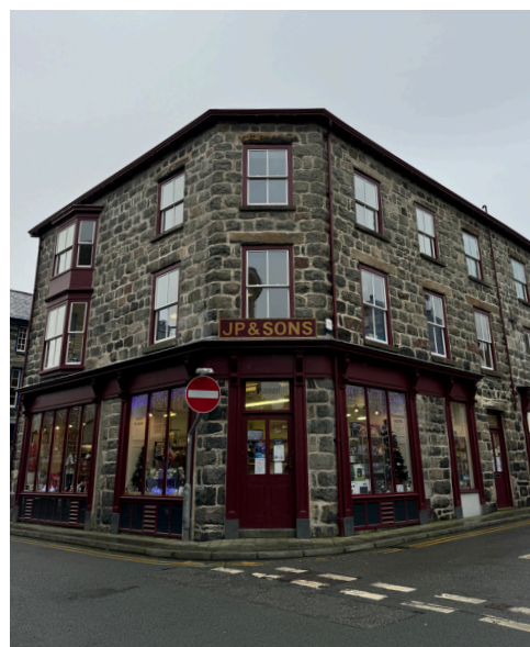
J P & Sons Shop, Dolgellau, renovated through the Dolgellau Townscape Heritage scheme
