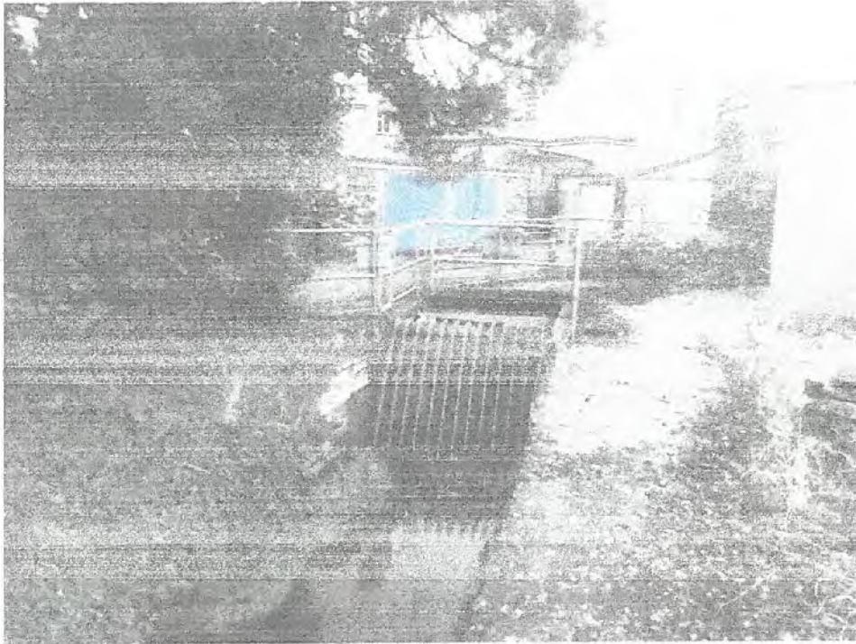
Photo 1. U/S Face main culvert beneath High Street, Penrhyndeudraeth
