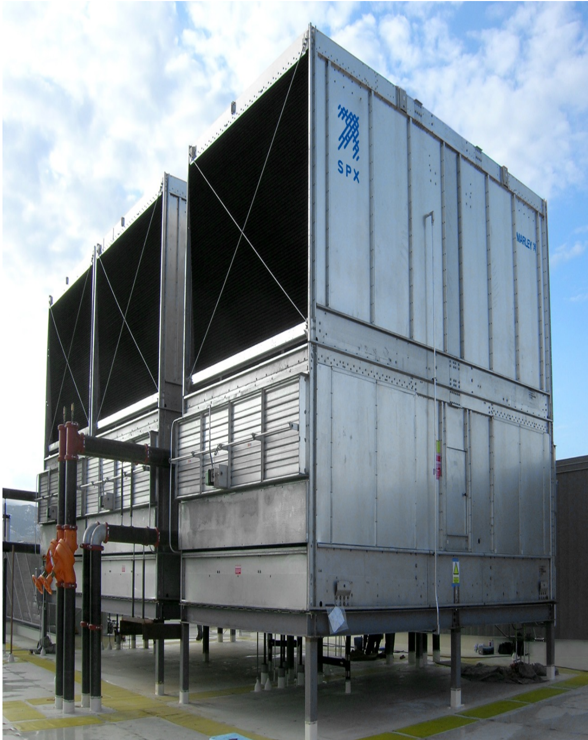
Figure 6.11 Indicative image of wet cell cooling towers
