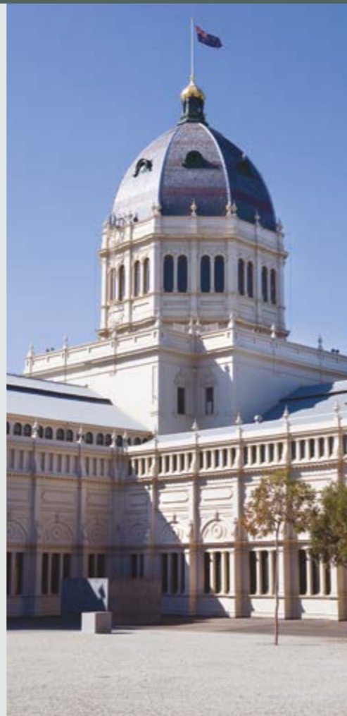
The dome of the World Heritage Royal Exhibition Centre in Melbourne (Australia) is covered in slate from Northwest Wales © Department of Environment (Australia).
